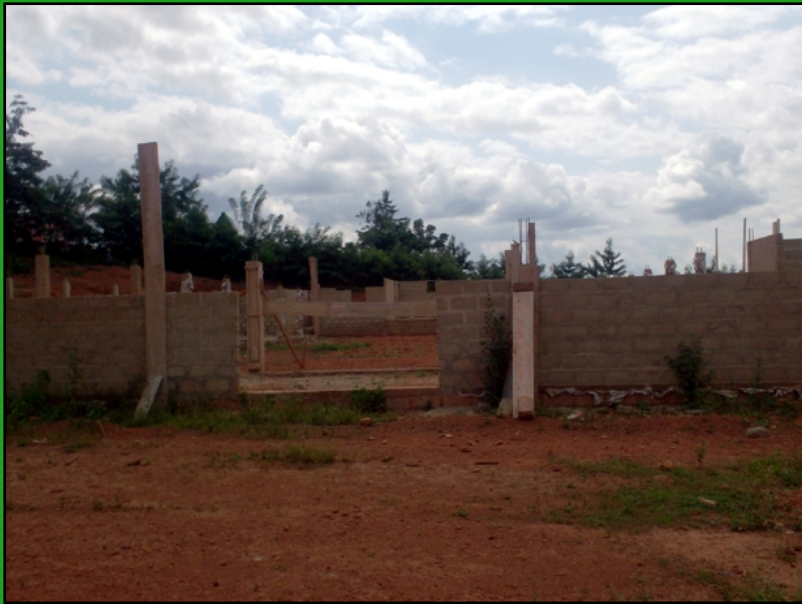
Yakase Community Center under construction
