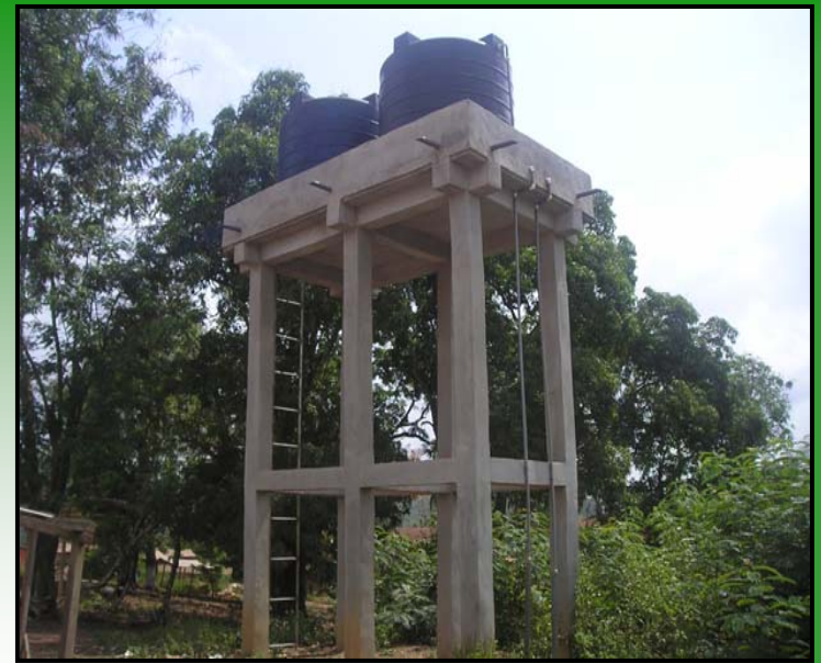
Abochia Borehole Mechanization
