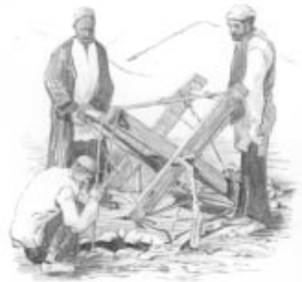
Figure 3 Muqannis Excavating Soil from a Qanat Shaft. Spoil lifted by windlass encircles the vertical shafts that link the qanat tunnel with the surface. Clearing blockage from qanat tunnels is usually required every few years. (Illustration by Ann Coffin Delano)
